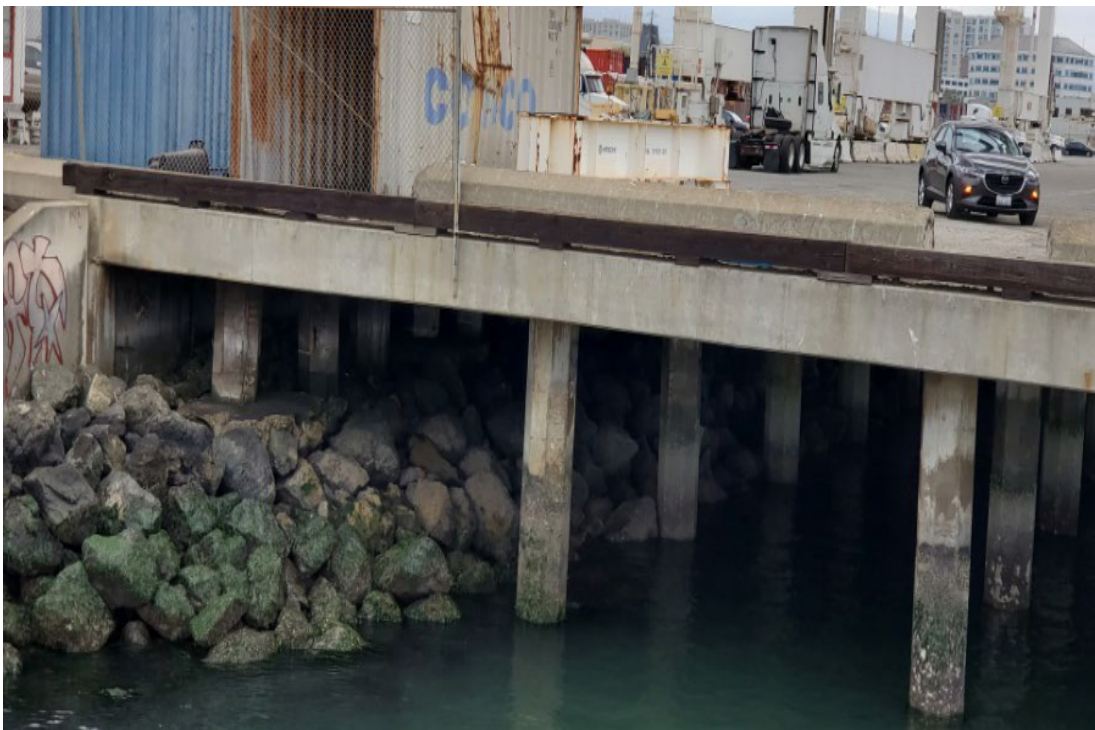
Figure 4. Typical Wharf Paving Deck Elevation, Howard Terminal
